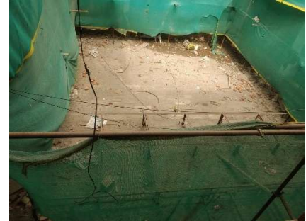
Fig 3.2. 6 Courtyard Source: Author
