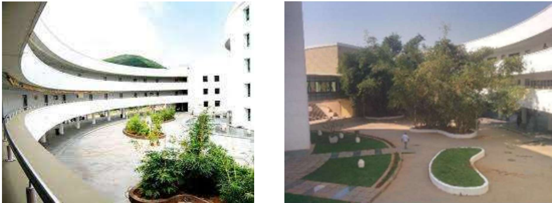
Fig 3.5 5 Block C (Left) and Outdoor Spaces (Right) Source: Help Arch
