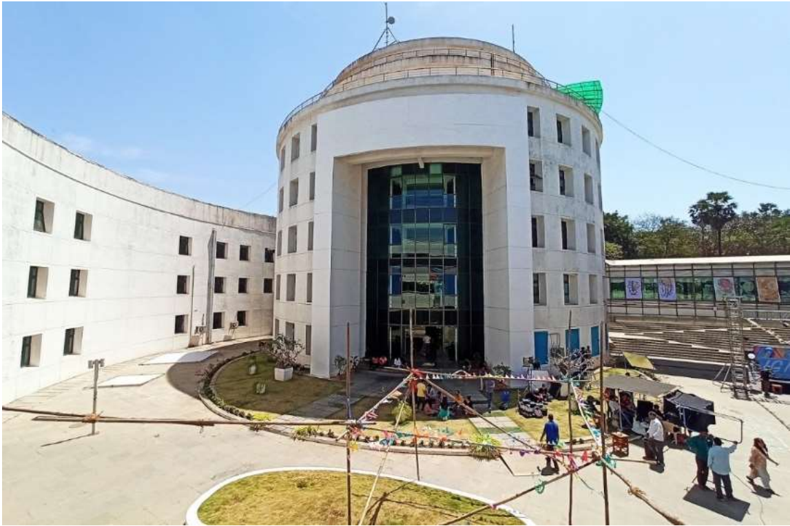
Fig 3.5 1 Exterior View of Institute Source: Shiksha
