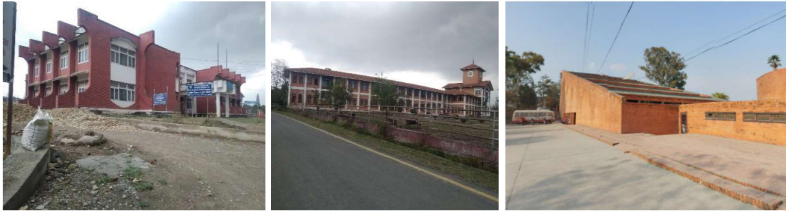
Fig 6. 8 surrounding building façade
