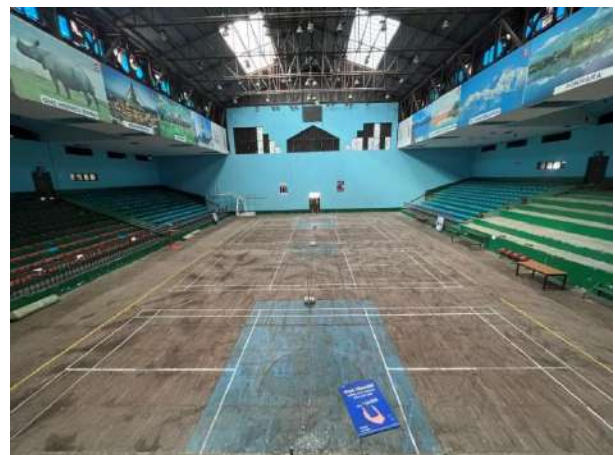
Figure 36: Court of Covered Hall
