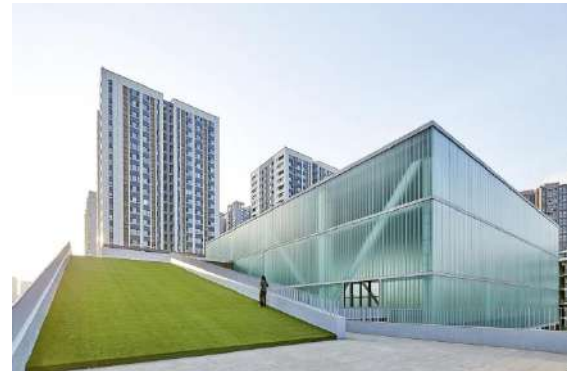
Figure 40: San Wayao Community Center, China
