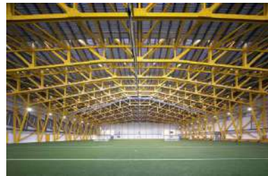
Figure 54: Steel Struss Structure
