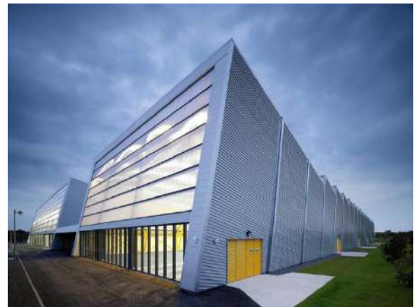
Figure 50: Ravenscraig Sports Facility
