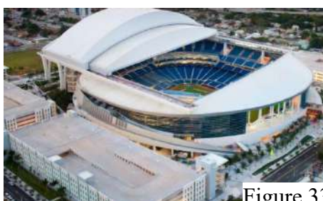
FIG: OPENED ROOF
