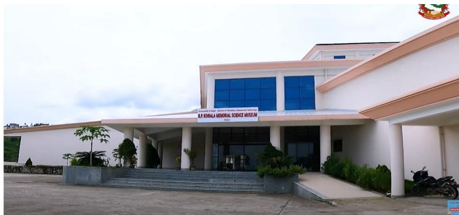
Figure: 46 entrance lobby
