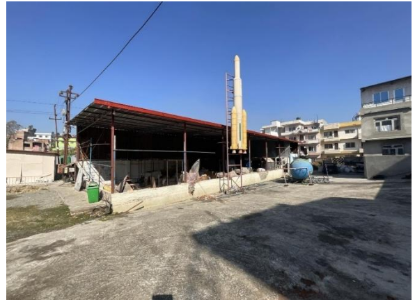
Figure: 48 abonded structure
