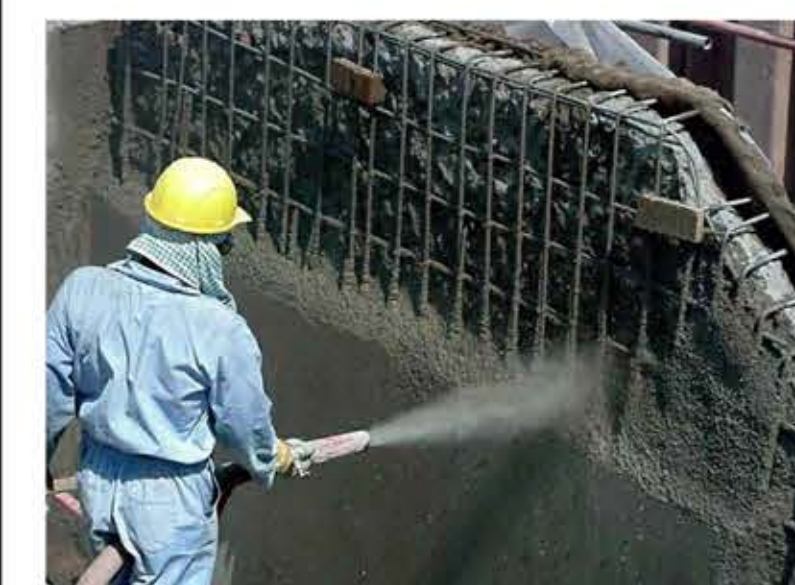
PILER WITH SHEAR WALL IN PLAZA
