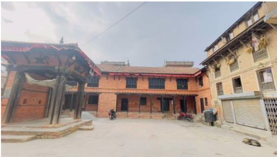
Figure 4.14 Showing open space courtyard
