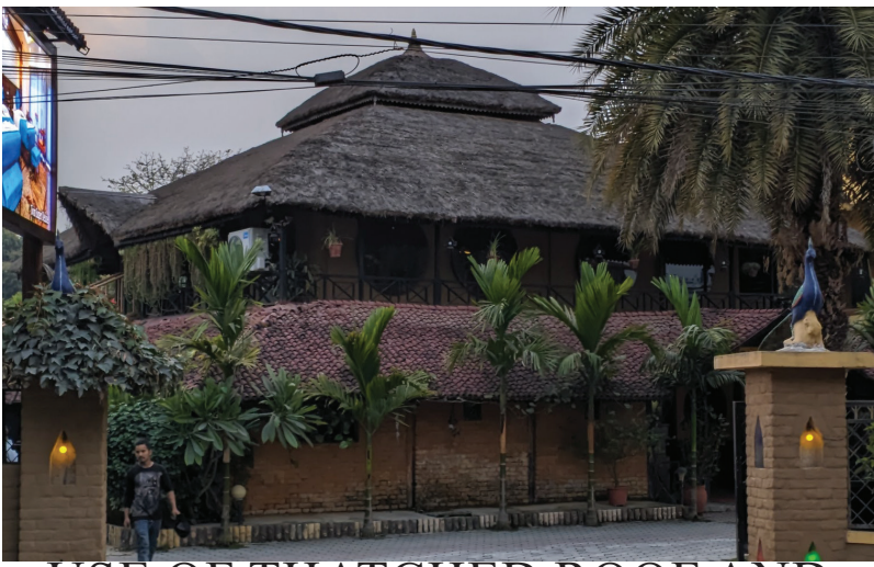
USE OF THATCHED ROOF AND WATTLE-DUB WALL OR MUD PLASTER
