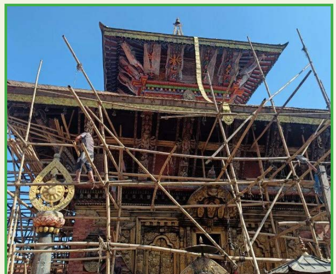
Renovation of Changunarayan Temple
