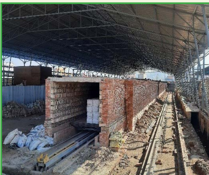
Local Brick Factory
