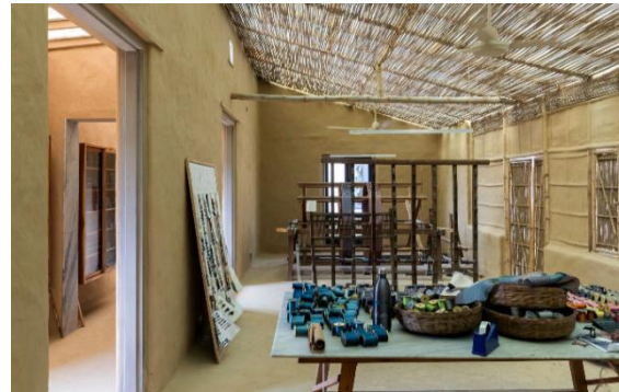
Figure 4.15: one of the workshop made with brick on walls and covered with lime.
