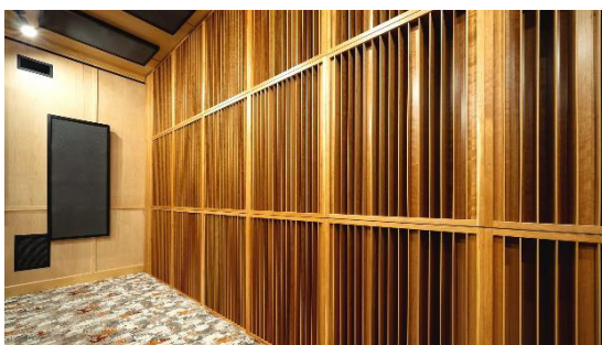
Fig2.32: Quadratic Residue Diffuser
