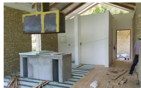
Figure 40 Insulation laying process on floor
