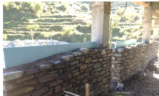
Figure 39 Insulation laying process on wall
