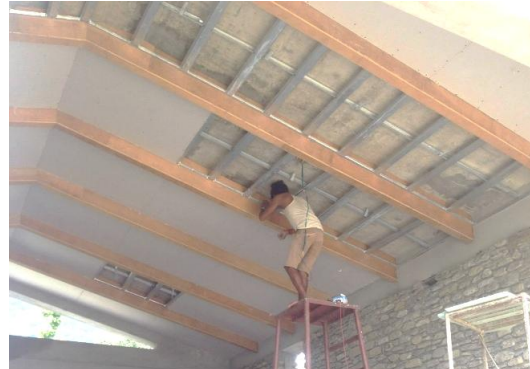
Figure 38 Insulation laying process on ceiling
