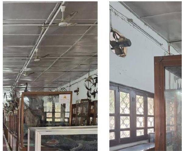
Figure 3.7: Ventilation through windows, ceiling fan and exhaust fan
