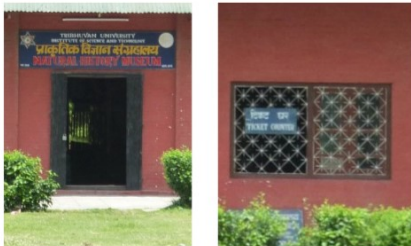
Figure showing channel gate and window grill
