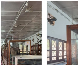
Fig showing ceiling and exhaust fan
