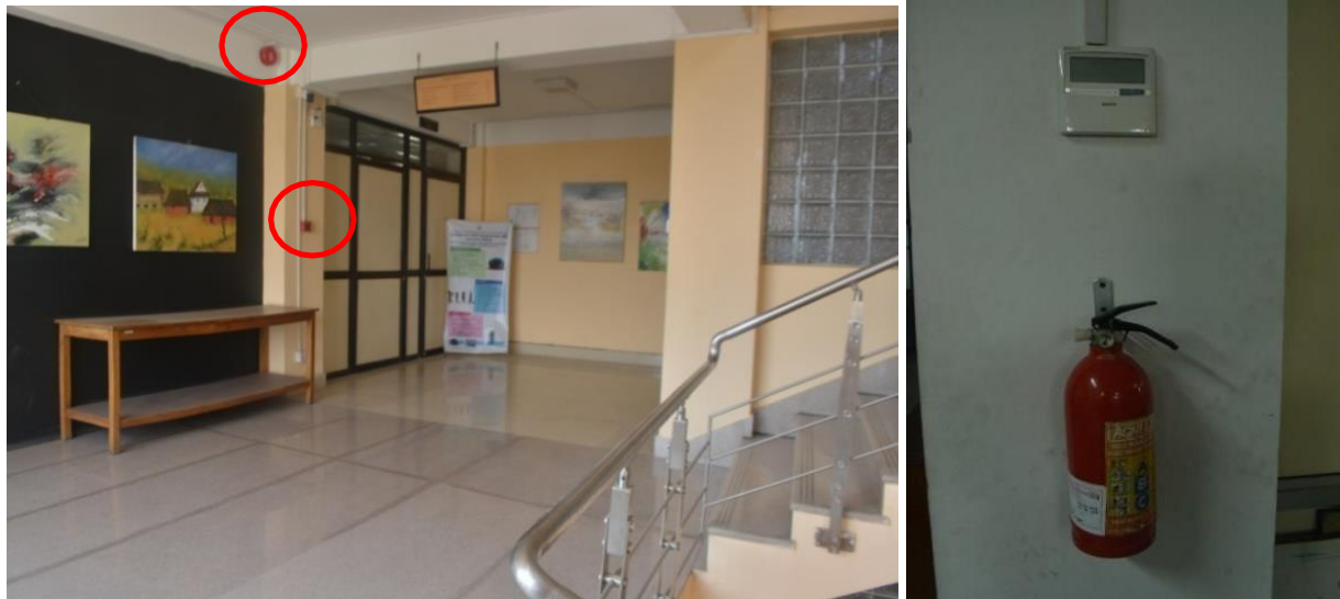
Fig 4. 20 : Fire extinguisher and fire alarms
